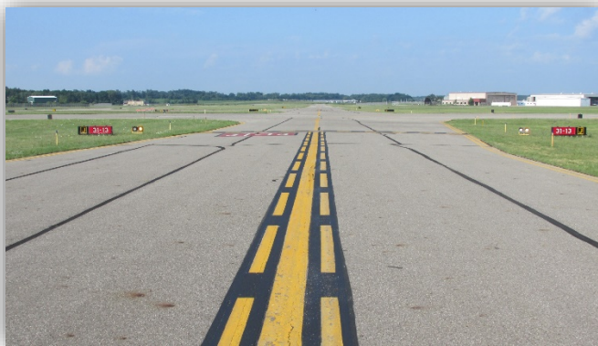
Enhanced Taxiway Centerline Markings
