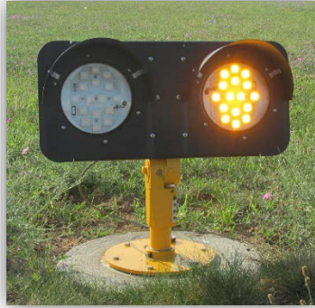
Elevated Runway Guard Light (RGL)
