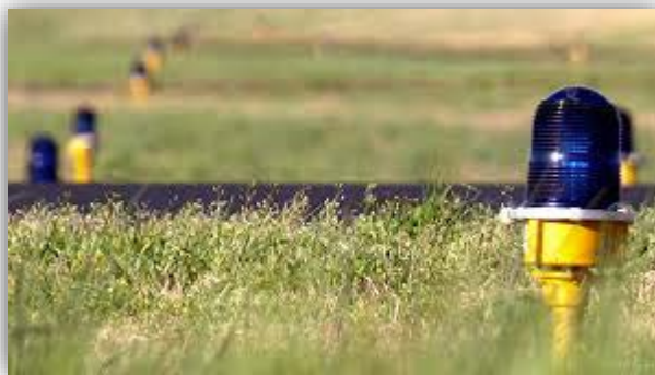
Taxiway Edge Light
