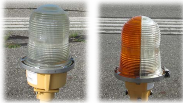
Runway Edge Lights
